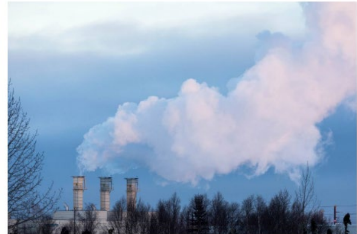
Exhaust from the Southcentral Power Project in Anchorage is lit by the setting sun on Friday, Jan. 11, 2019. (Loren Holmes / ADO)
