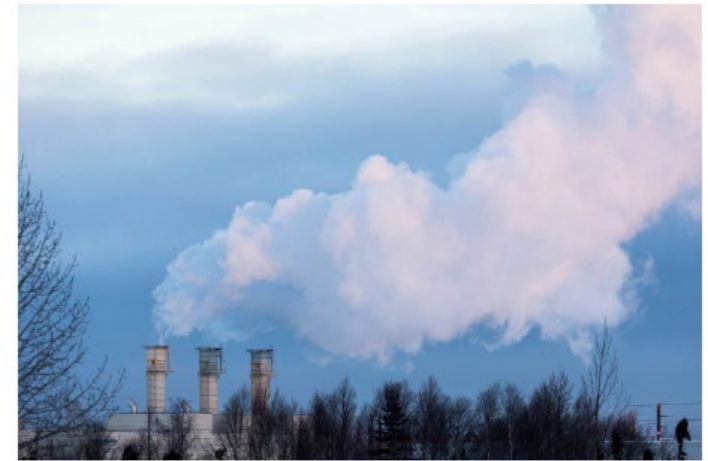
Exhaust from the Southcentral Power Project in Anchorage is lit by the setting sun on Friday, Jan. 11, 2019. (Lorenz Holness / ADN)
