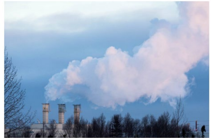
Exhaust from the Southcentral Power Project in Anchorage is lit by the setting sun on Friday, Jan. 11, 2019. (Lorenz Holness / ADN)
