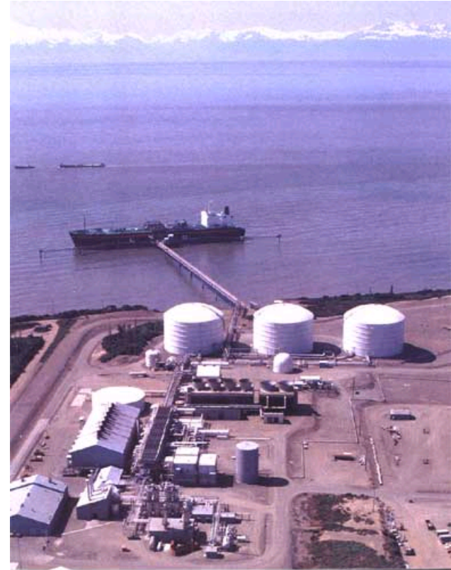
Kenai Export Terminal, Alaska Photo courtesy of CH-IV International, http://ch-iv.com
