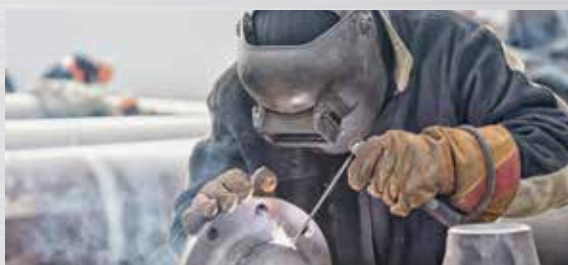
Welders – Fabricate and assemble metal structures and pipelines.
